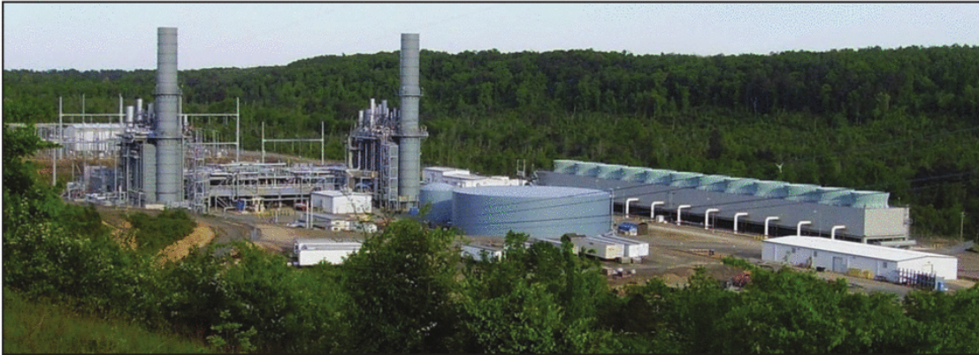
The Hot Spring, Texas, U.S.A., combined-cycle power plant of Suez Energy Generation North America has implemented the Commander software by AAT for the optimization of its start-up procedure.
