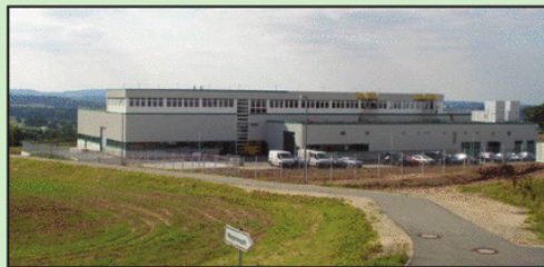
The new production facility of MTS Deutschland located in Bayreuth, Germany, is for the manufacture of gas turbine blades.
